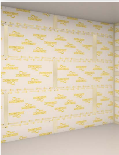
7._ Vertical joints 2nd layer
