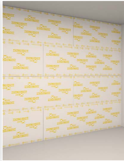
2._ Boards installed horizontally
